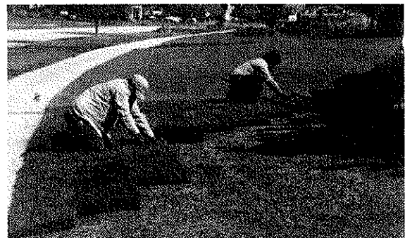
Figure 5. Sodding produces an instant lawn.
